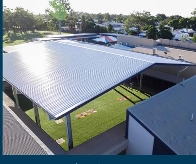
From Tender Concept to For Construction, our engineers were able to refine the steel design, by shaving a little over 2T of steel and approx. ~\$12k off our tender price, delivering a more economical build for the Client. Access was very tight and MSE designed the structure in a way that the Roof could be assembled in the carpark and lifted in one lift meaning Structural Steel Erection only took 3 days to complete allowing other trades to get in and complete their works on time.
